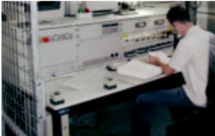
Computer-aided, high-voltage test equipment ensure tested quality
