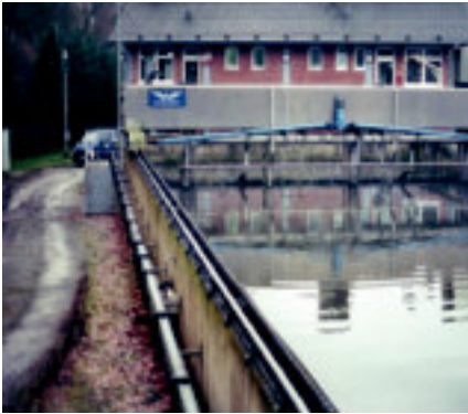
The scraper moves on the 38 m long final clarifier in round-the-clock operation. The energy supply is done via the LBT Flizz® system
