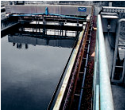
LBT Flizz® in a longitudinal scraper travel (S) = 38 m ● Speed (v) = 1.0 m/min. ● Acceleration (a) = 0.5 m/s 2 ● Cycle time 1.5 x hour/ 24 h/365 days
